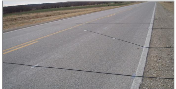
**Set up of Road Tubes Sensors for Data Collection on Vehicles' Lateral Position**
